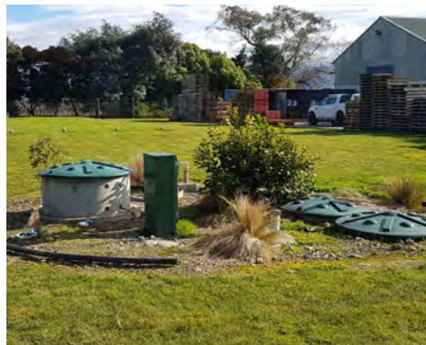
Example of a site-scale wastewater management system.
