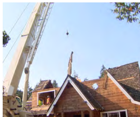
Example of a home being deconstructed.
