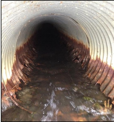
Figure 2. Lake Ida Ann Drain Culvert
