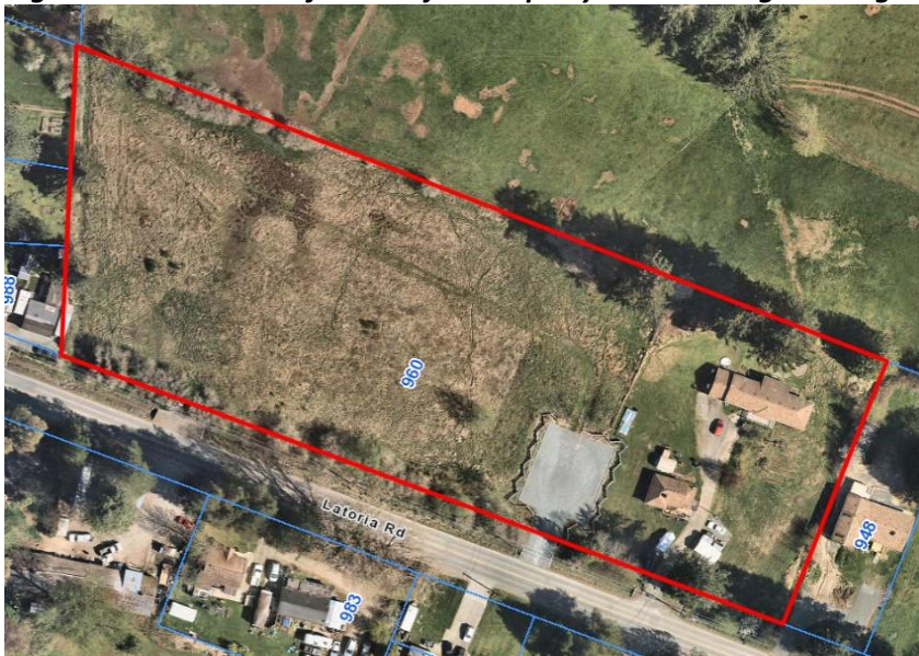
Figure 1: Aerial View of the Subject Property with Existing Buildings and Structures
