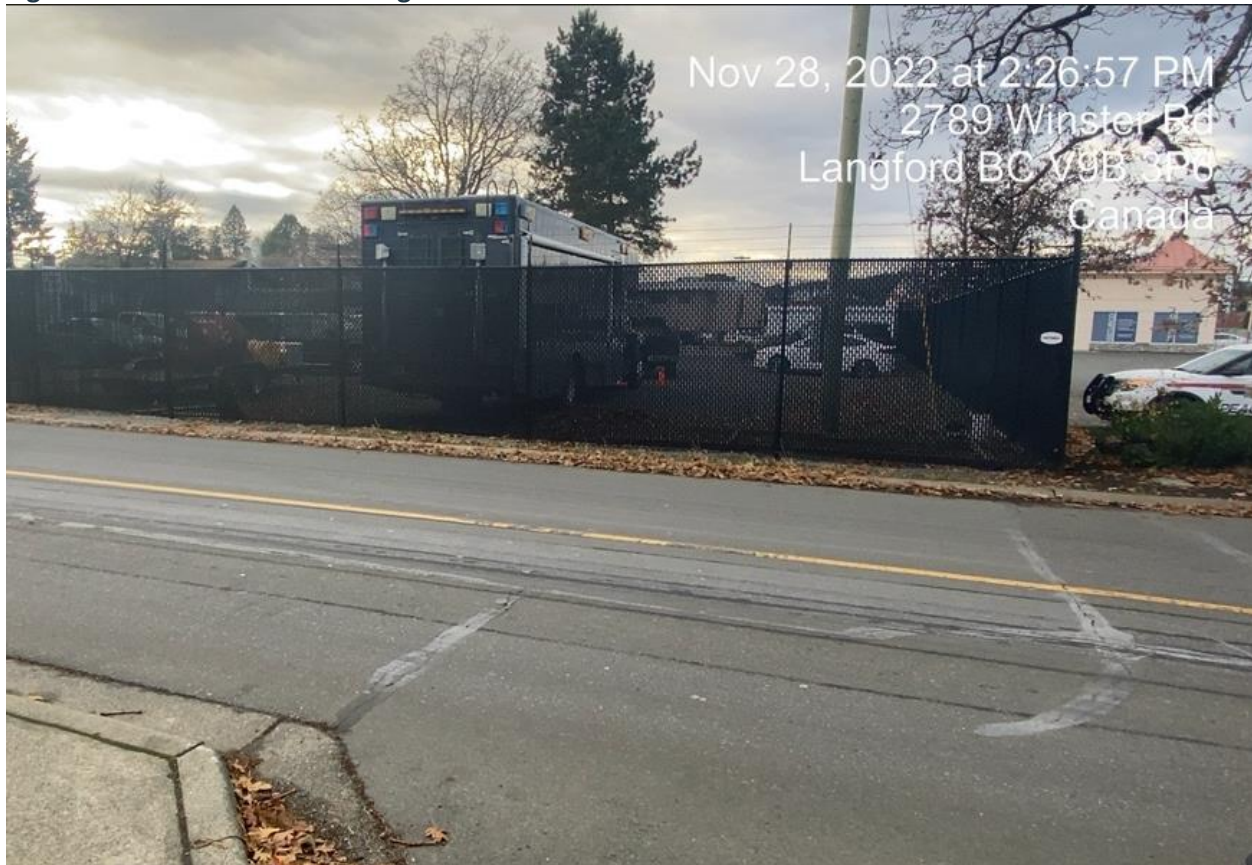
Figure 1: New Chain Link Fencing
