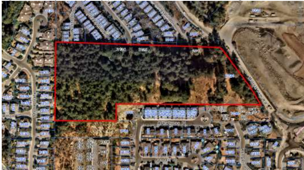
Figure 1 – Subject Property (image does not reflect site clearing that has since occurred)
