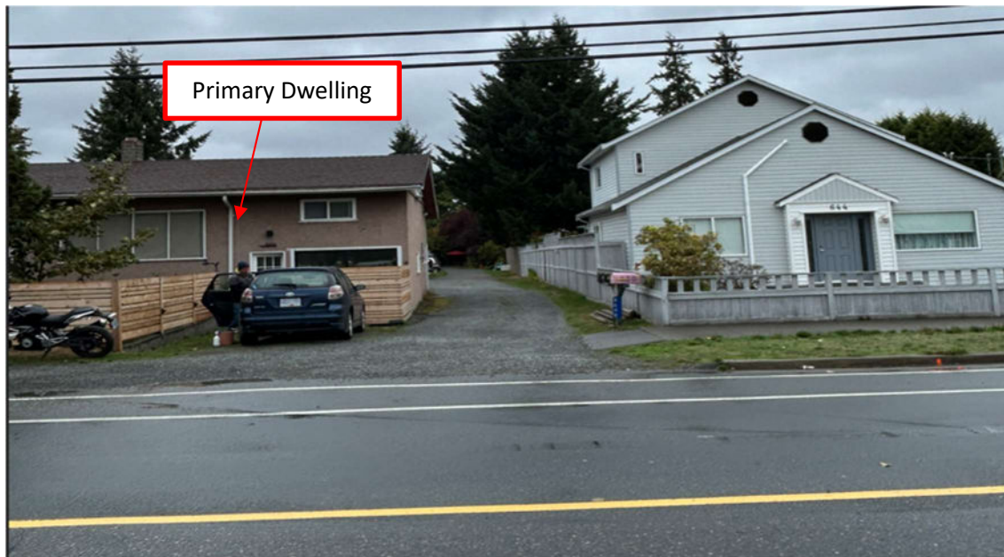
Figure #2 –Site Photo- NW view of driveway. Atkins Ave frontage.
