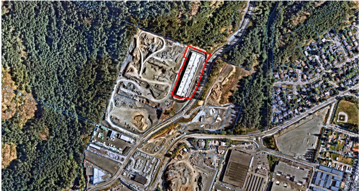
Figure 1: Subject Property and Surrounding Neighbourhood
