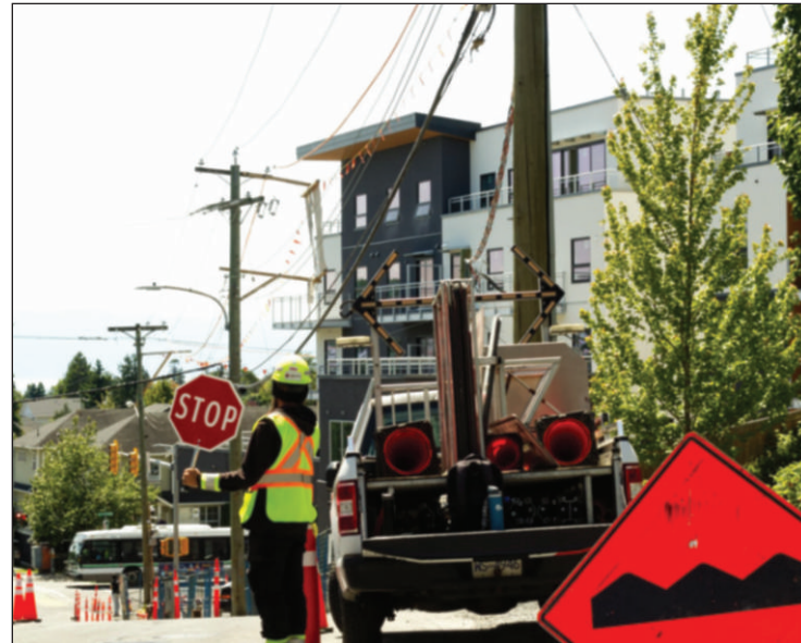
Esquimalt has surpassed the province's one-year housing targets after just six months. (Evan Lindsay / Black Press Media)
