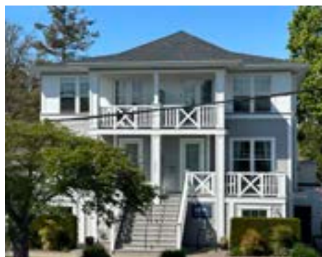
Example of a three storey multi-plex.
