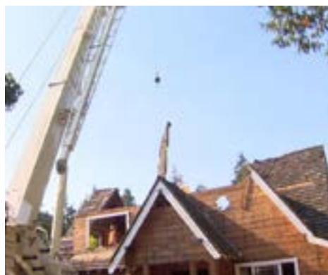
Example of a home being deconstructed.
