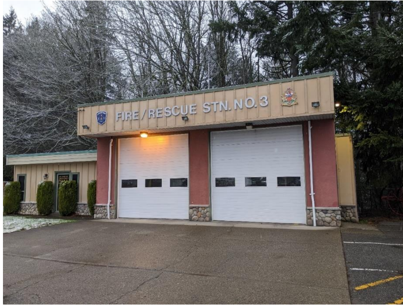
Photo 6 City of Langford Fire Rescue Station 3.
