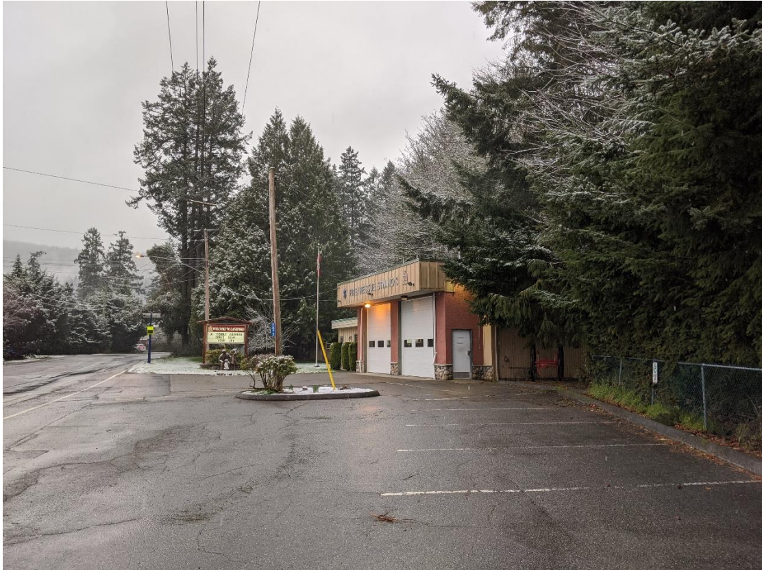
Photo 13: Power lines adjacent to forests are sources of ignition as trees or branches fall onto the lines.
