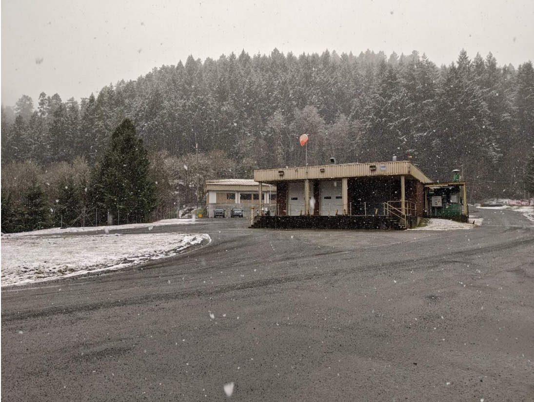
Photo 7 CRD water disinfection facilities at Japan Gulch.
