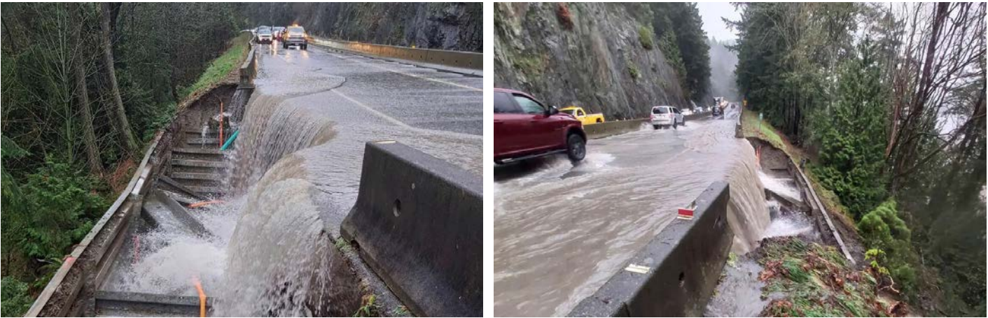
Landslide on the Malahat (2021). Photo credits: Emcon Services
